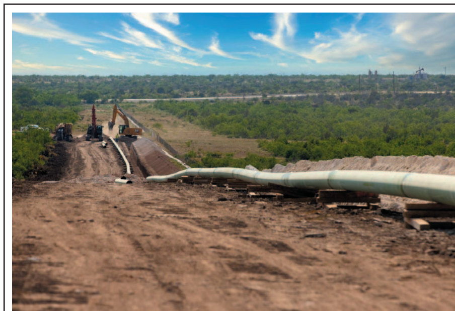
In the Midland Basin, Brazos Midstream is building more than 70 miles of large diameter, high-pressure gas gathering pipelines to address constraints in parts of Reagan, Glasscock, Midland and Upton counties. The company says its pipeline expansions and improvements will maximize flow assurance, reduce fuel and line loss and ultimately improve producer net backs.
