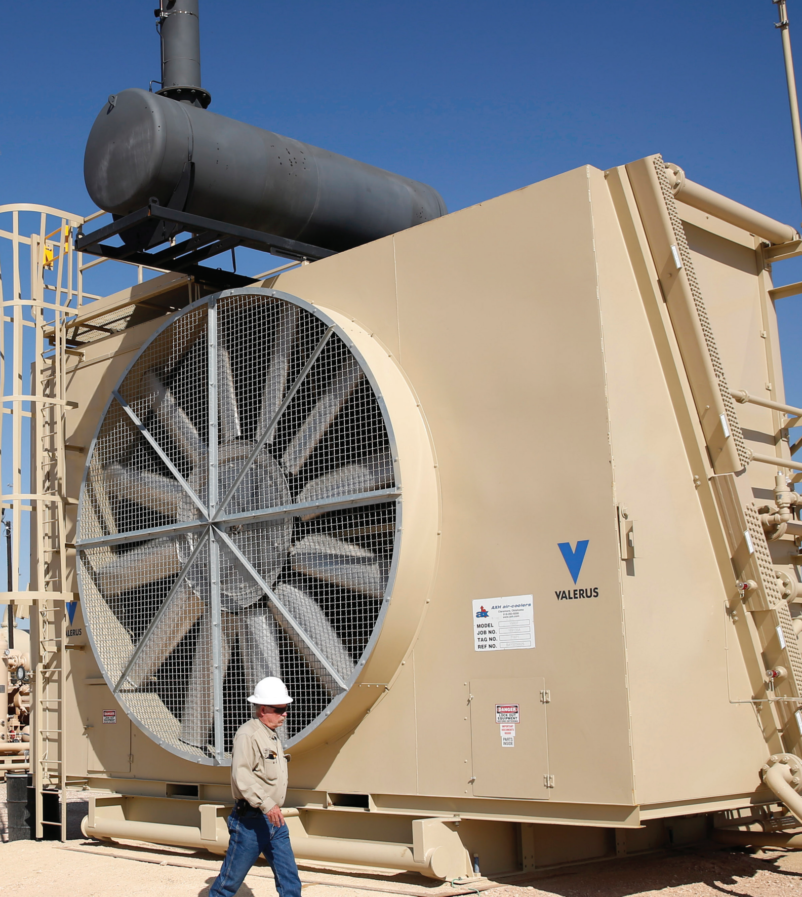
Brazos Midstream's Robert Hollander inspects a row of compressor units at the Miller Compression Station servicing Delaware Basin producers near Barstow, Texas.
